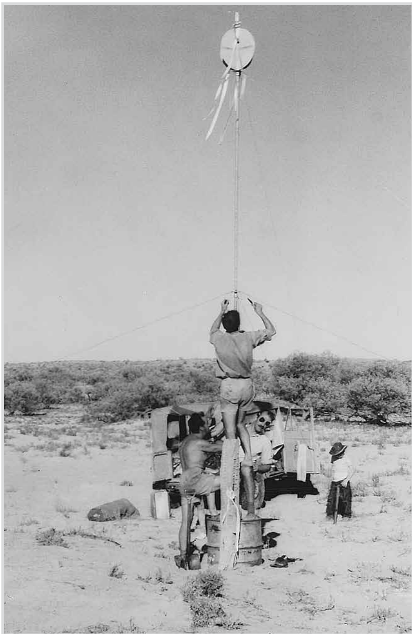
Erecting the Geosurveys 'trig' station, Poeppel Corner, 1962.
